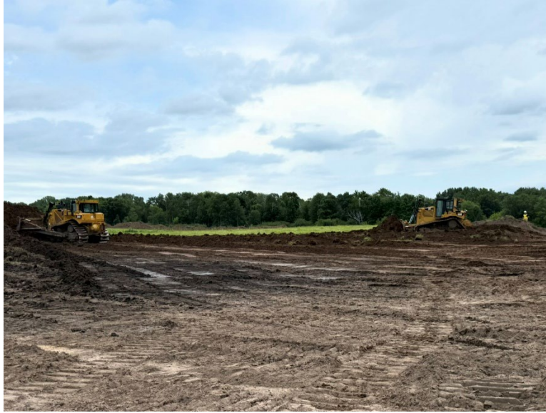
Facing south near MP 0.2, view of contractor stripping topsoil
