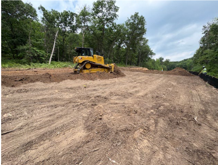
Facing east near MP 2.35, contractor continues topsoil segregation
