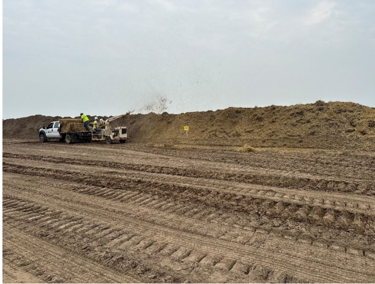
Facing east near MP 1.8, view of contractor seeding and mulching stockpiles
