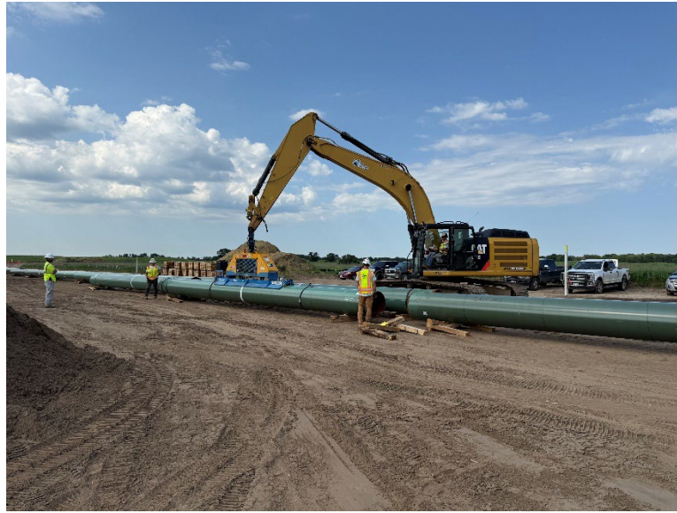
Facing east near MP 1.76, view of contractor stringing line pipe
