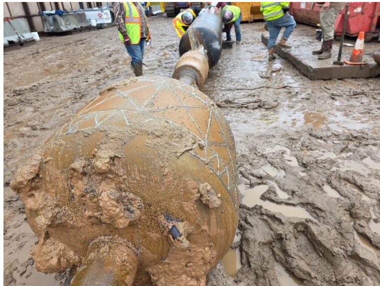
HDD P4-3 completed the pull
