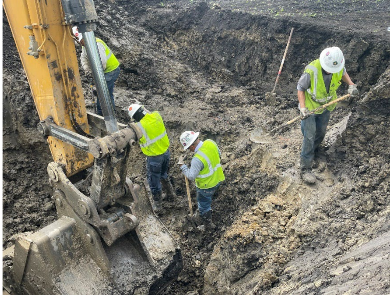
Facing southwest at MP 31.1, K&K excavating line stop location for the MNM80105 E-line south of 135th Street
