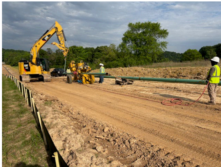
Facing southeast near MP 3.0, contractor bending branch line pipe
