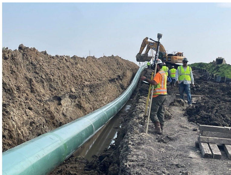
Facing south at MP 33.9, K&K lowering-in mainline pipe
