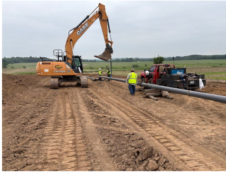
Facing west near MP 3.4, contractor stringing bore pipe
