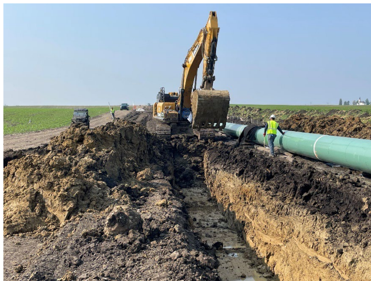
Facing south at MP 33.7, K&K trenching for mainline pipe
