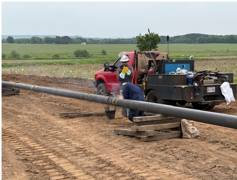
Facing south near MP 2.95, contractor welding bore pipe
