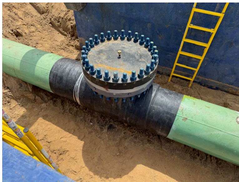
Near MP 1.0, line-stop flange installed
