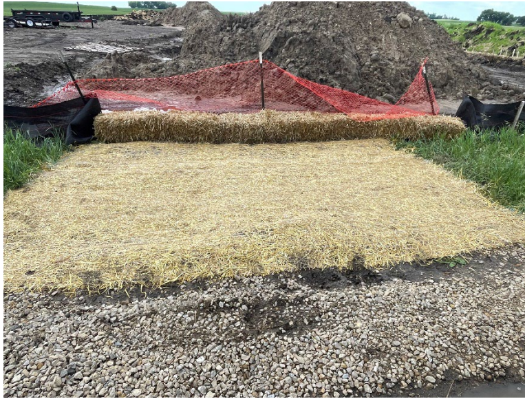
Facing south at MP 34.15, ECBs installed for 165th Street south bar ditch
